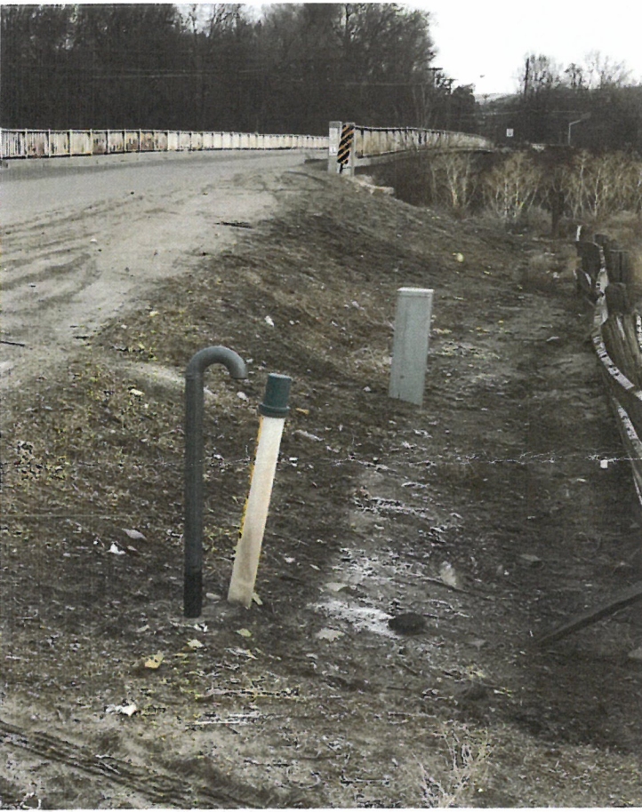
Figure 4: Vent Stack for Casing 26701305
