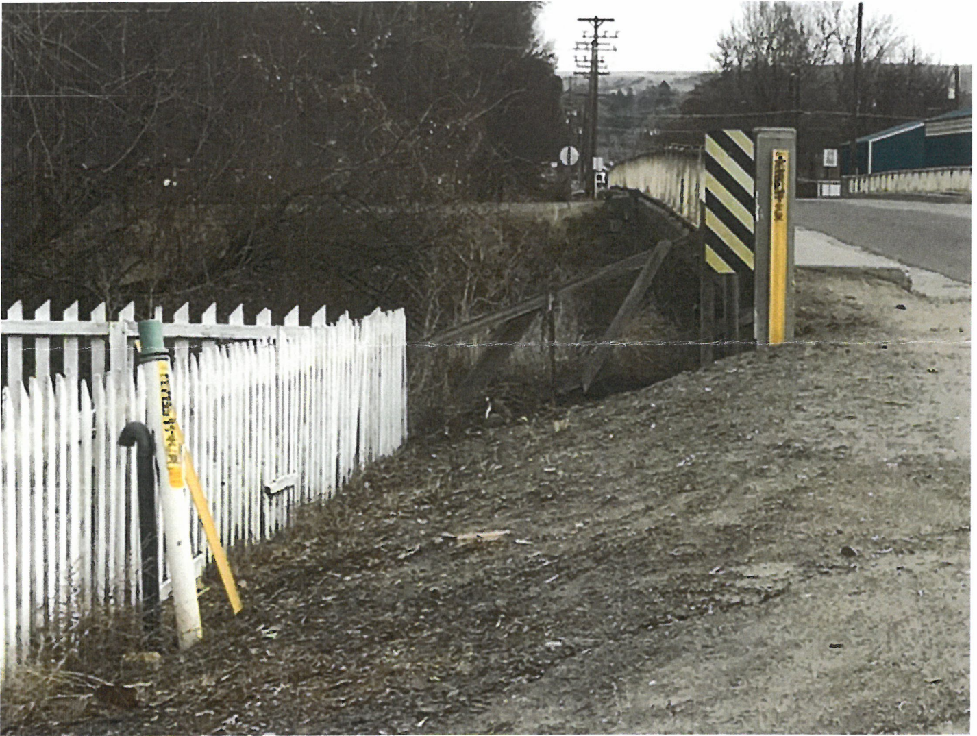
Figure 1: Vent Stack for Casing 26701315
